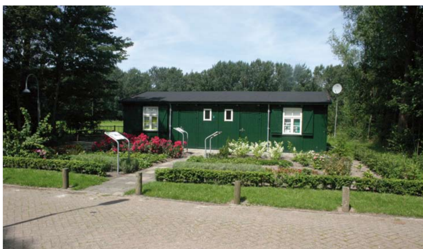
Barak in Tollebeek
